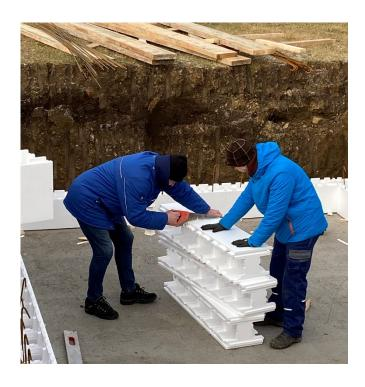
Next, drill an 8mm (=every 50cm) hole in every second chamber of the base plate - this is for the vertical reinforcement. We recommend cutting the 8mm bars to a length of 150cm and inserting them into the holes provided. If you take the 150cm bars, the vertical reinforcement is already finished and you do not need to tie a short piece of bar every second layer. If you assume a pool depth of 150cm, the 150cm long irons will fit perfectly. (10cm into the brine and 140cm outside the bottom plate).
